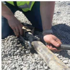
Tighten with two wrenches.
