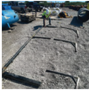
Layout the bottom corners.
