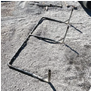
Attached the bottom corners.
