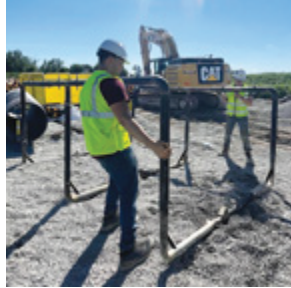
Add bottom corners then second top section.
