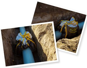
Installation is safe and simple. Fill the PipeSak® weight with aggregate from a local source; distribute along the right of way; lower over the pipeline; and back-fill. PipeSak's can be installed with a single lift hook and can be released without workers in the trench.
