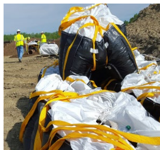
Transport to stockpile.
