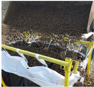
Evenly fill with ballast.
