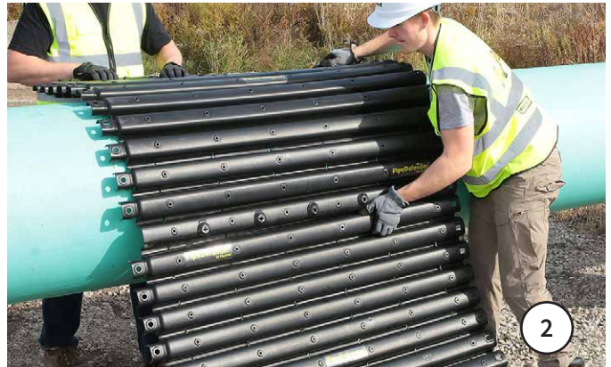
Drape panels over pipe. Attach additional panels as required for pipe diameter.
