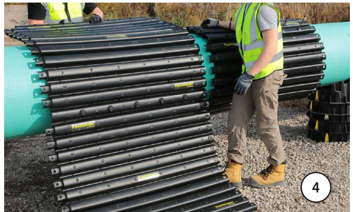
Lay next panel set OVER the teeth of the first section, overlap ridge and fasten.
