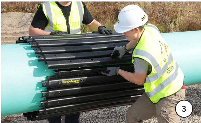
Attach panels overlapping ridge and fasten (4 QuickZip fasteners).
