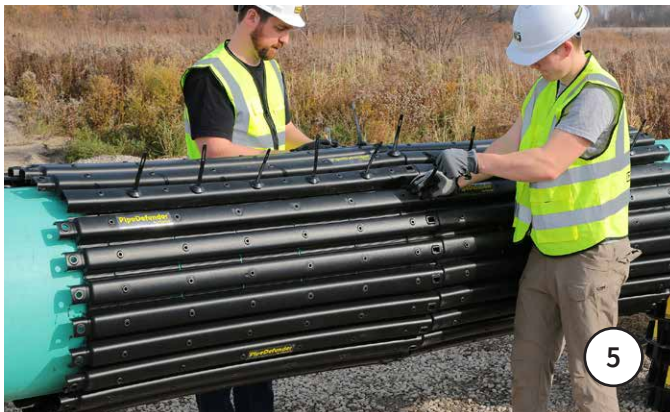
Fasten two panel sets together (circumference) with 8 QuickZip fasteners. Trim off excess QuickZip.
