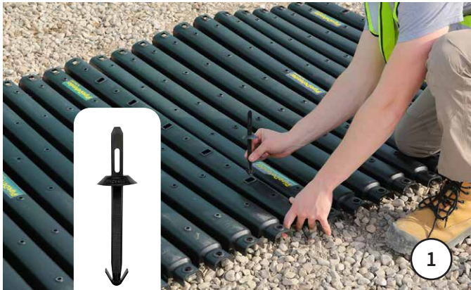
Prepare fasteners and panel sets of two for specific pipe diameter (4 QuickZip fasteners).
