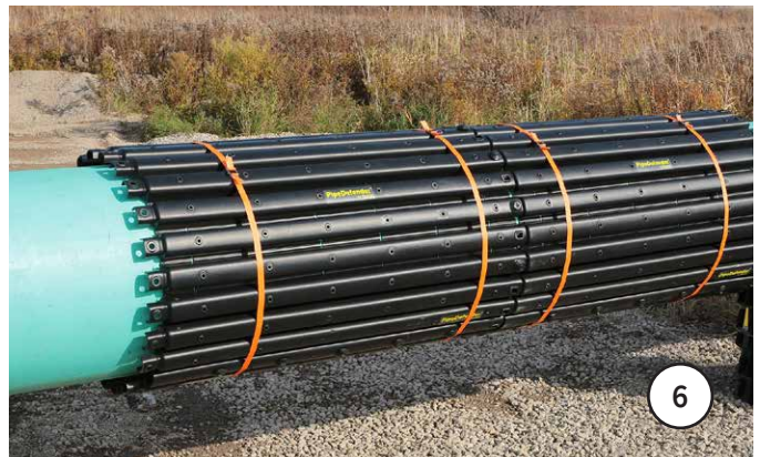
As panels are completed, add strapping to secure (2 straps per panel set).
