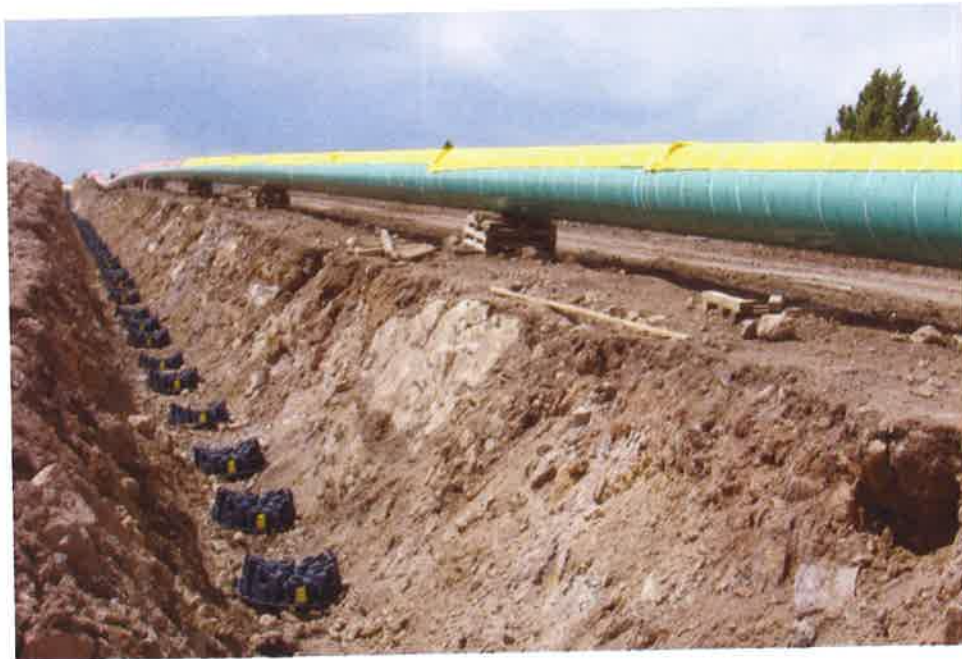
Figure 8. SPP in trench.
