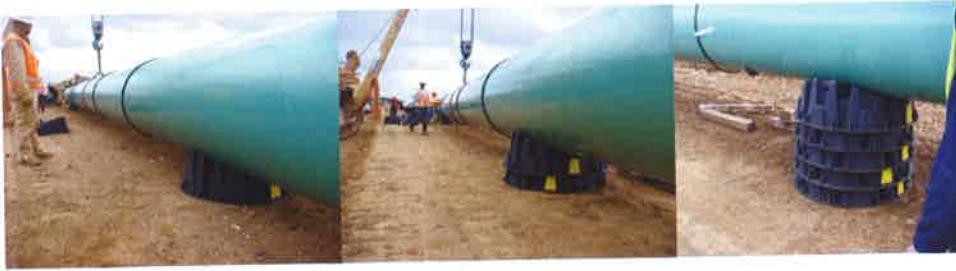
Figure 7. SPP skid replacement outside of trench.
