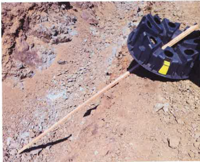
Figure 9. SPP installation in trench.
